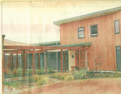
Well clad: The Schoenberg home from the south entry, showing the lawson cypress shiplap cladding.
