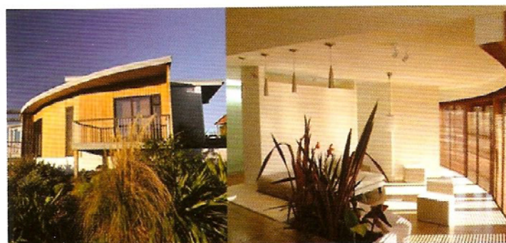
Left: Sunlight and shadow in this semi-circular house demonstrate the benefits of passive solar design for winter sun and summer shade. Right: A sunken living room allows higher windows and sunlight to enter deeper into the building in winter.
