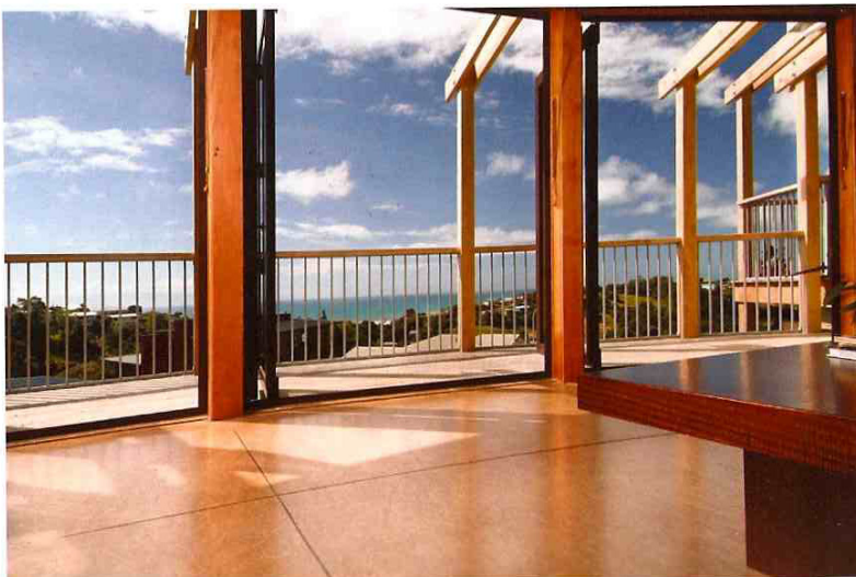
Thermal mass exposed
