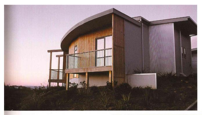
▲► Economical yet effective: the Nelson home of architect Helen Richards, of Powered Living, maximises passive solar design. North-facing windows act as solar collectors, while concrete internal walls store and gradually release the heat. This approach to design makes a lot of sense, and is certain to become more widespread as the cost of energy becomes of increasing concern.
